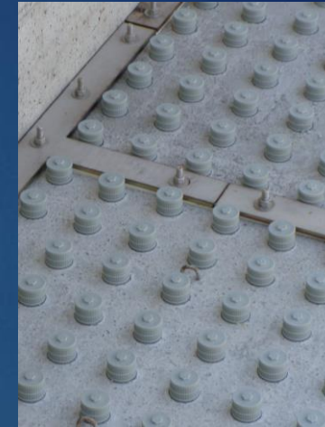
Nozzles Floor Installed
