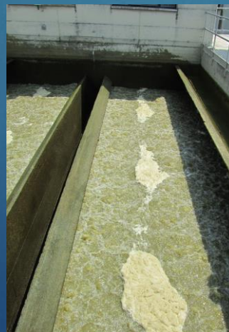
Gravity Filter Air Backwash
