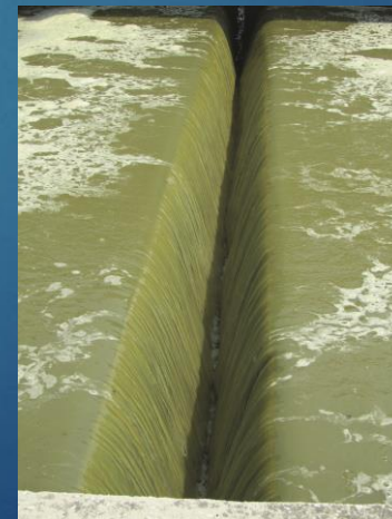
Gravity Filter Water Backwash
