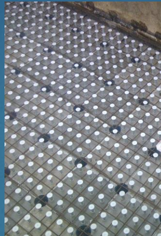
Nozzles Floor under construction
