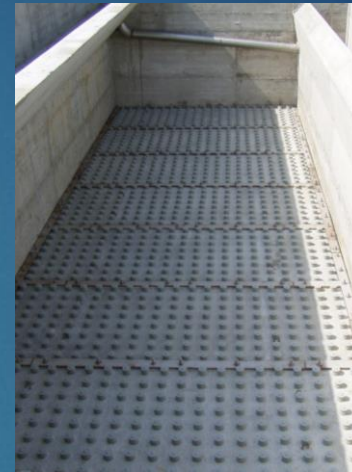
Nozzles Floor Installed
