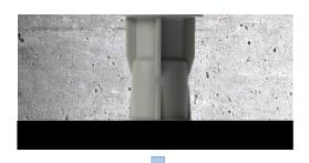
Check the sleeves! All sleeves should be perfectly levelled in the whole floor
